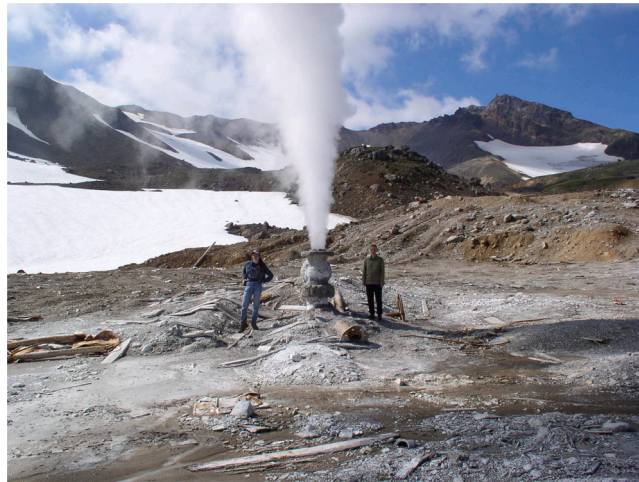
Photo-1 Blowing well 035 at the foothills of Mutnovsky volcano (see Fig. 2 for well location). Photo by A. Kiryukhin, 2005. Unbearable noise around this well and significant reduce of wellhead saturation temperature (down to 80 °C at atmospheric pressure) was observed here since 2017.
