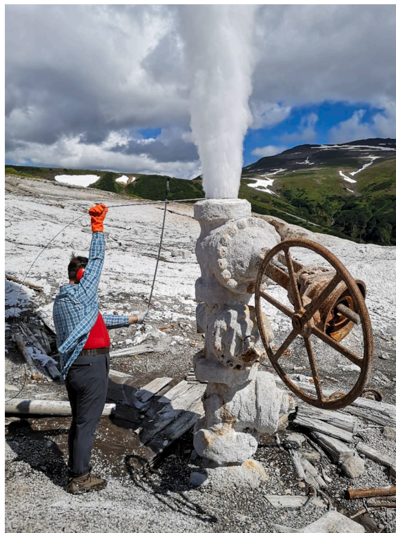
Photo-1 Blowing well 035 at the foothills of Mutnovsky volcano (see Fig. 2 for well location). Photo by A. Kiryukhin, 2005. Unbearable noise around this well and significant reduce of wellhead saturation temperature (down to 80 °C at atmospheric pressure) was observed here since 2017.
