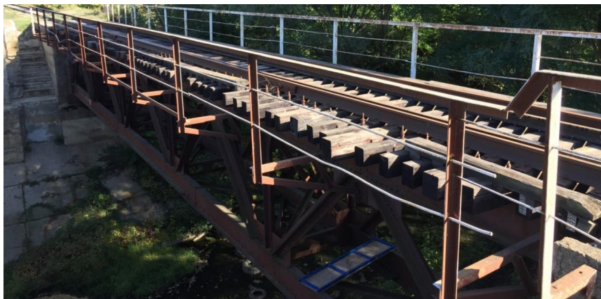
Fig. 1. General look of the bridge
