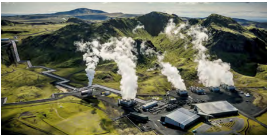
Hellisheiði geothermal power plant owned by Reykjavík Energy, Iceland. Carbfix
