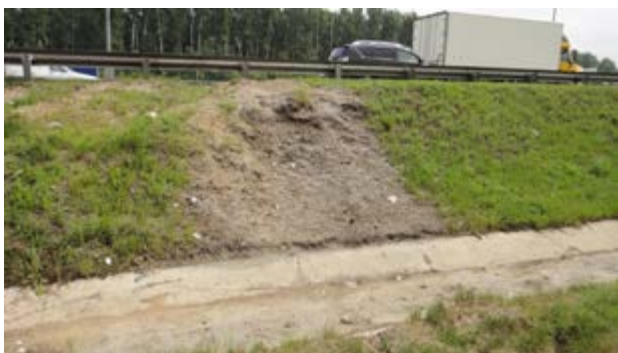
Pic. 1 The place of tanker accident
