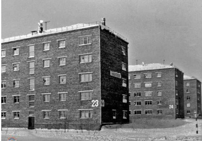
Figure 1. Typical residential house in Igarka. Image 1: In 1983 (five years after construction). Image 2: In 2011 (33 years after construction). Note significant permafrost-related structural deformation in the second photograph.
