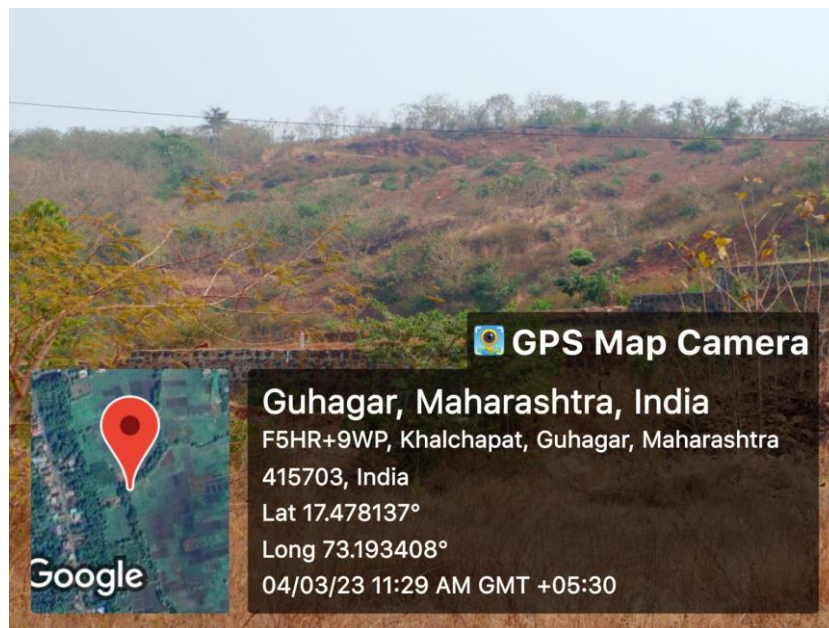
Field Photograph 3. Excavation of topsoils in the study area which prove the decreasing the planation and increase urbanisation which lead to decrease the groundwater recharge which will effect the quality of water in terms of increase the salinity ingress in natural
