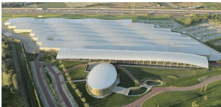
Figure 1. Technogym headquarter in Cesena, Italy (source: Arketipo).
