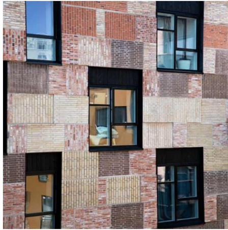
Figure 1. Patchwork façade of the Resource Rows residential complex built with masonry panels from the deconstruction of the Carlsberg Brewery, Copenhagen, Denmark. Photo by Mikkel Strange. Source https://www.theguardian.com/cities/2020/jan/13/the-case-for-never-demolishing-another-building
