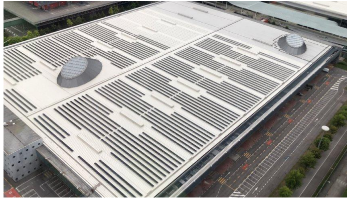
Figure 2. Fiera Milano exhibition centre (Rho-Pero, Milano, Italy) pavilions provided with roof-top tilted photovoltaic modules strings.
