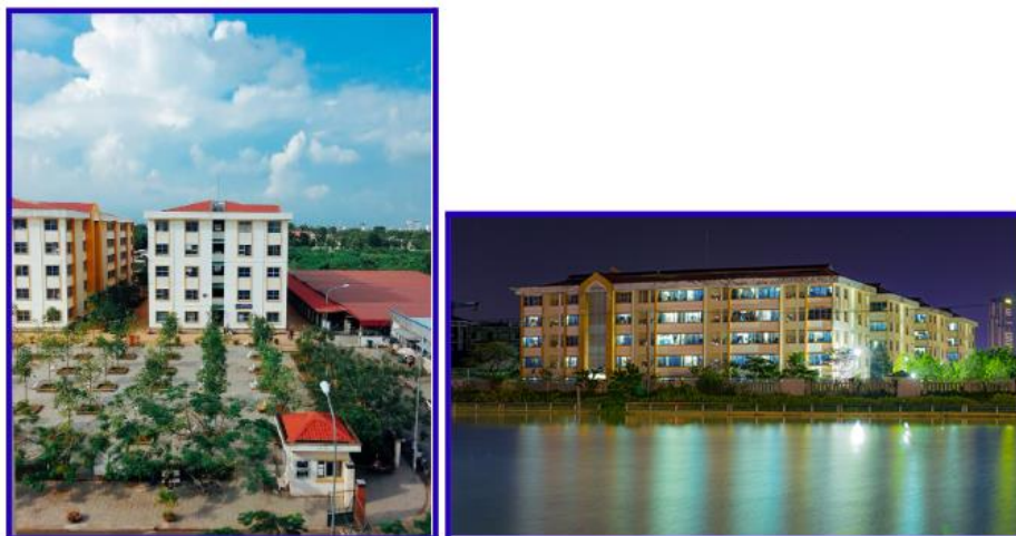
Figure 5. New Construction of A Residential Area for Can Tho University Staff
