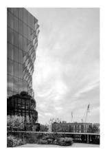
Studio Gang, the Chicago-based architecture firm, designed the 139,000-square-foot building using a strategy it describes as "solar carving." The architects mapped the sun's annual course to determine which parts of the nearly finished 12-story tower to slice away and sheathed portions of those sections in tilted angular panes of glass.
