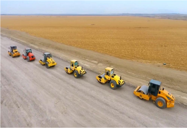
Pic 1. The construction of the Ahmadbeyli-Horadiz-Minjivan-Aghbend highway in Azerbaijan.
