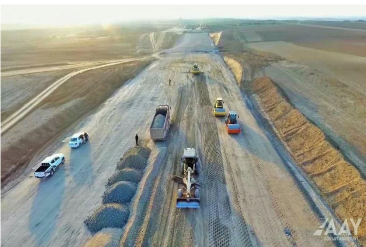
Pic 3. The construction of the Ahmadbayli-Fuzuli-Shusha highway.
